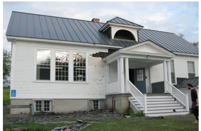
The new metal roof, looking all spiffy in July.
