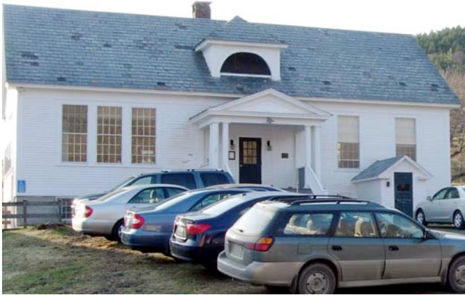
Our patchwork slate roof earlier in the spring.
